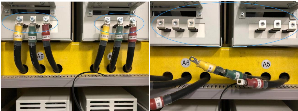
(Step1: Power cell Input terminal)
