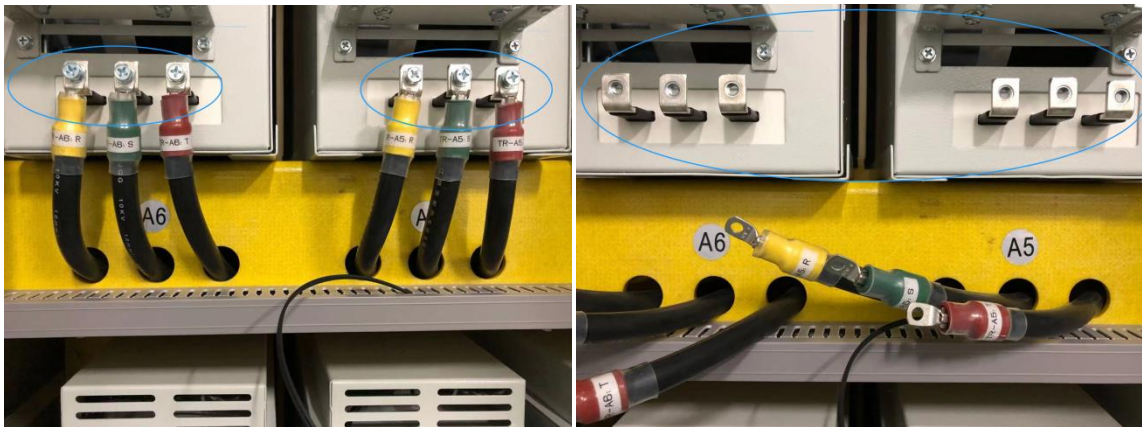
(Step1: Power cell Input terminal) (單元輸入端)
